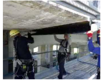
Work using conventional methods
