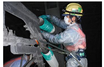
Conventional paint application work
