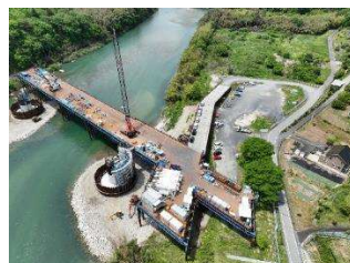
No. 2 Kiso River bridge caisson construction
