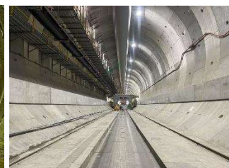
Metropolitan Tunnel No. 1 (Kajigaya Section) Full-scale excavation
