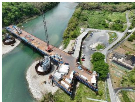
No. 2 Kiso River bridge caisson construction
