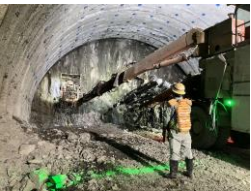
Osashima Tunnel Excavation of main shaft
