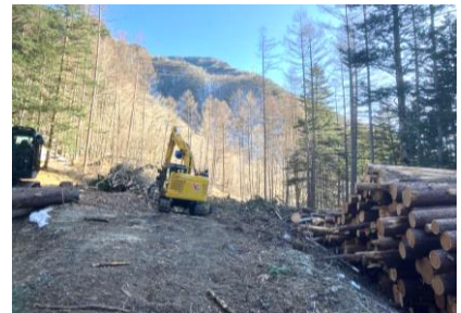
Preparatory work for the yard (tree cutting)
