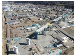
Ajima North Viaduct
