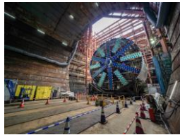
Metropolitan Tunnel No. 2 Shield machine assembly completed
