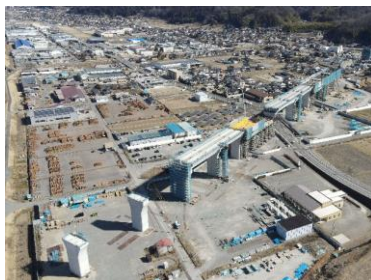
Ajima North Viaduct
