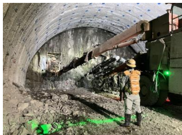
Osashima Tunnel Excavation of main shaft
