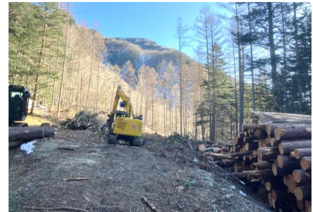
Preparatory work for the yard (tree cutting)
