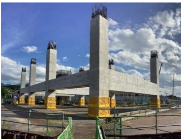
Gifu Prefecture Sta. (tentative name) Elevated bridge
