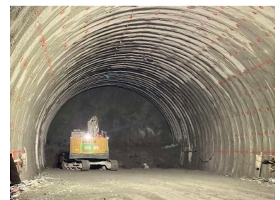
Southern Alps Tunnel (Yamanashi Section) Excavation of main shaft
