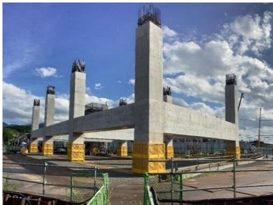
Gifu Prefecture Sta. (tentative name) Elevated bridge
