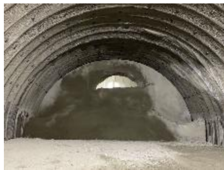
Progress of main shaft excavation for Inasanchi Tunnel (Tochu/Mibusawa section)
