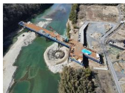
No. 2 Kisogawa Bridge Pier Foundation work
