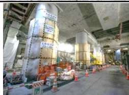
Shinagawa Station (Trenchless construction section) Excavation under the rail
