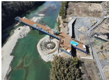
No. 2 Kisogawa Bridge Pier Foundation work
