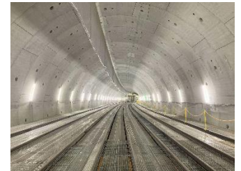
Metropolitan Tunnel No. 1 (Kitashinagawa Section) Survey tunneling completed
