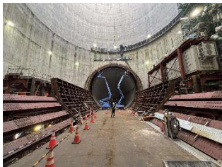
Chukyo Area Tunnel No. 1 (Sakashita west section)
