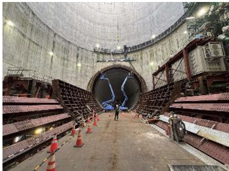
Chukyo Area Tunnel No. 1 (Sakashita west section)
