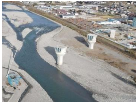
Bridge railing on the Tenryu River Pier construction
