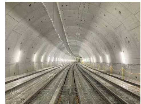
Metropolitan Tunnel No. 1 (Kitashinagawa Section) Survey tunneling completed
