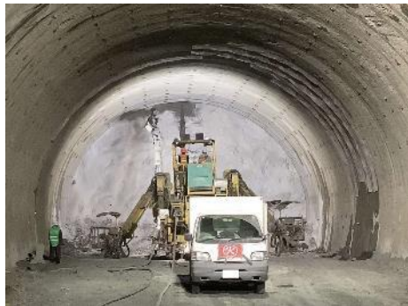
Minamikoma Tunnel No. 4 (East section) Excavation of main shaft
