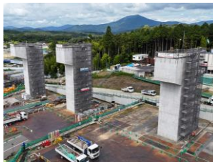
Gifu Prefecture Station (tentative name) Deadhead line pier work
