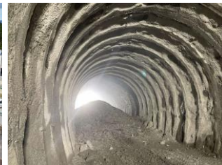
Southern Alps Tunnel (Nagano Section) Pilot tunnel penetration (Nozokiyama Emergency Exit - Kamazawa Emergency Exit)
