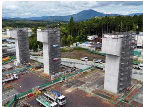
Gifu Prefecture Station (tentative name) Deadhead line pier work
