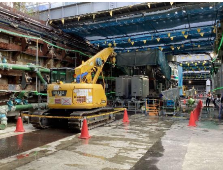
Nagoya Station (Central East Section) Diaphragm wall (excavation)
