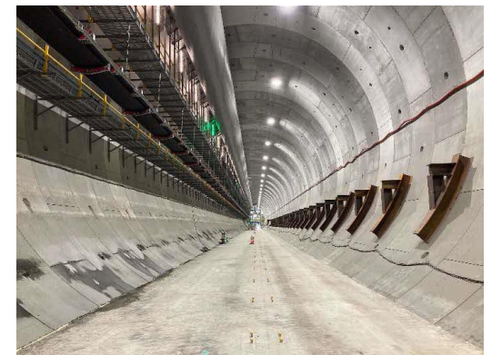
Metropolitan Tunnel No. 1 (Kajigaya Section) Full-scale excavation
