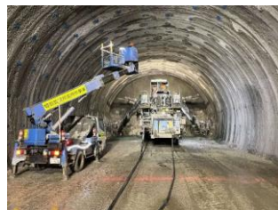
Inasanchi Tunnel (Tochu/Mibusawa section) Excavation of main shaft
