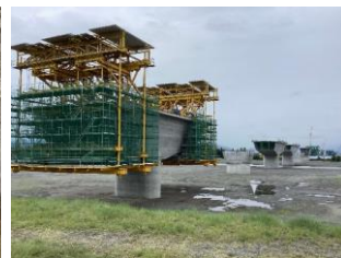
Bridge railing on the Kamanashi River Superstructure
