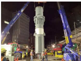
Nagoya Station (Central west section) Construction of a pillar of the underground station building
