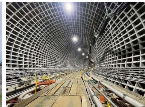
Metropolitan Tunnel No. 1 (Kajigaya section) Full-scale excavation
