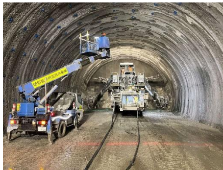
Inasanchi Tunnel (Tochu/Mibusawa section) Excavation of main shaft
