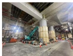
Excavation under the rail at Shinagawa Station
