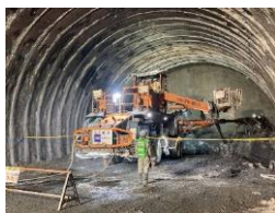
Southern Alps Tunnel (Yamanashi section) Excavation of main shaft
