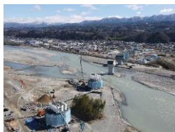
Construction of piers of bridge railing on Tenryu River
