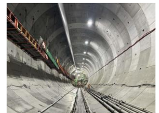
Metropolitan Tunnel No. 1 Kajigaya section Inside the shaft
