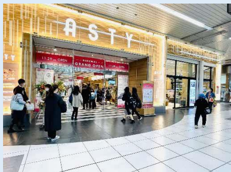
Renovation of ASTY Shizuoka (West Building)
