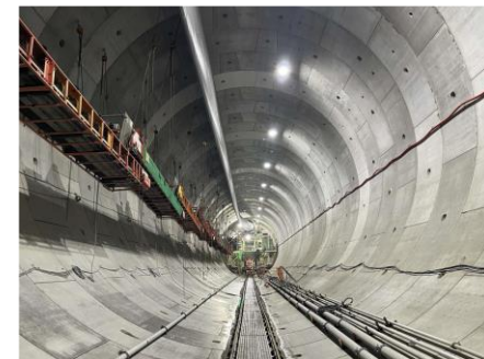
Metropolitan Tunnel No. 1 Kajigaya section Inside the shaft
