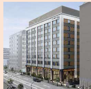
Appearance image of Courtyard by Marriott Kyoto Station (scheduled to open in FY2026)
