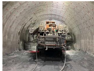
Southern Alps Tunnel (Nagano Section) Excavation of main shaft
