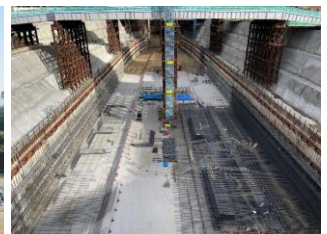
Kanagawa Prefecture Station (tentative name) Reinforcement
