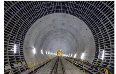
Tokyo Metropolitan Area Tunnel No. 1 Higashiyurigaoka construction area
