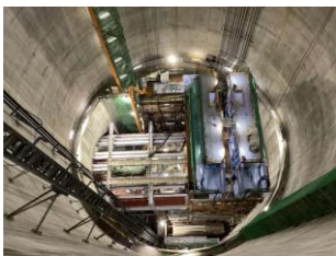
Chukyo Area Tunnel No. 1 (Meijo Section) Shield tunneling preparation
