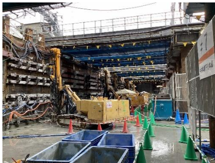
Nagoya Station Central East Section chemical injection (excavation)
