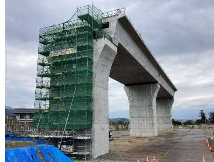
Tonegawa Park viaduct
