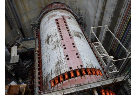
Metropolitan Area Tunnel No. 1 Kajigaya section survey tunneling
