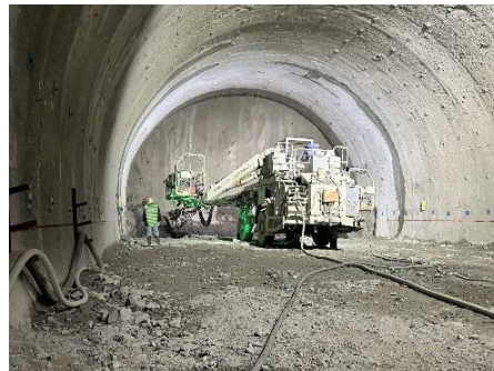
Seto Tunnel excavation of main tunnel
