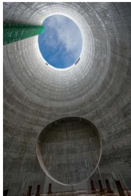
Jinryo Emergency Exit Completion of main vertical shaft
