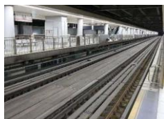
Shinagawa Station Completion of girder bridge for construction
