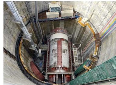
Metropolitan Tunnel No. 1 Kajigaya Section Status of shield machine
