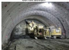
Chukyo Area Tunnel No. 1 Omori Section Excavation of main shaft
