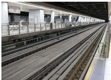
Shinagawa Station Completion of girder bridge for construction
