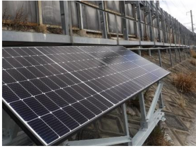
Solar power generation on Shinkansen banking (test installation)
