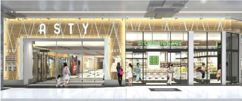
Renovation of ASTY Shizuoka (West Building)
