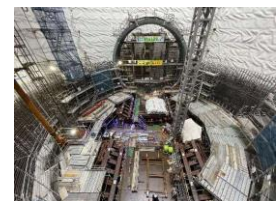
Higashiyukigaya Emergency Exit Construction of framework
