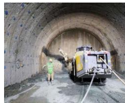
Fujino Tunnel in Kanagawa Prefecture Excavation of main tunnel
