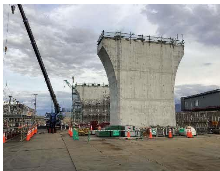
Usuiwara elevated bridge in Yamanashi Prefecture Construction of pier
