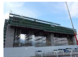
Elevated bridge in Yamanashi Prefecture Upper structure construction work
