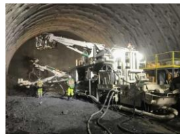
Southern Alps Tunnel Nagano Section Excavation of main tunnel
