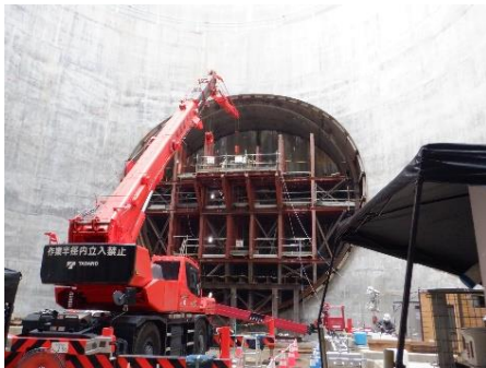
Chukyo Area Tunnel No.1 (Meijo Section) Preparatory work for shield tunneling
