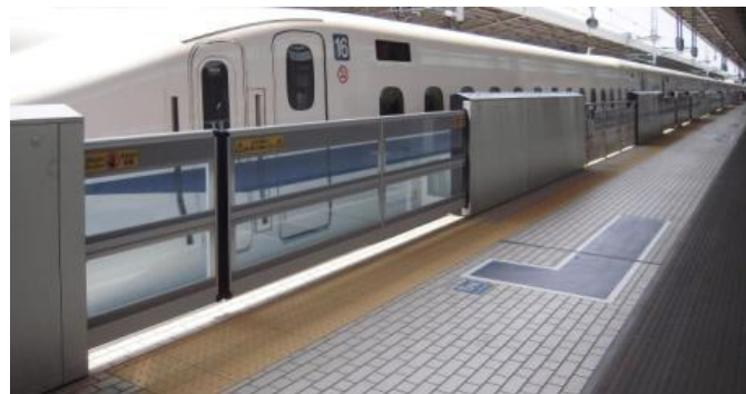
Install platform doors at all Tokaido Shinkansen stations
