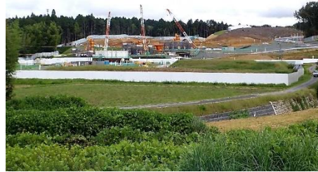
Gifu Prefecture Station (tentative name) Whole view of the railyard
