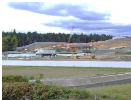
Gifu Prefecture Station (tentative name) Whole view of the railyard
