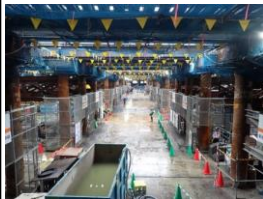
Nagoya Station Central East Section Excavation below train track
