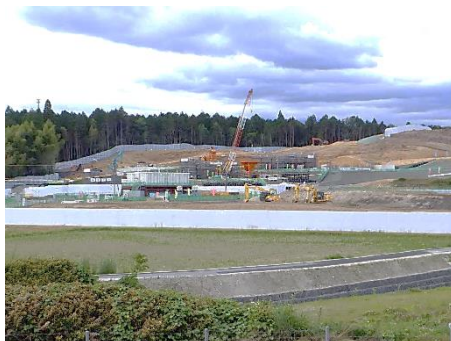
Gifu Prefecture Station (tentative name) Whole view of the railyard
