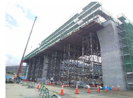
Viaduct in Yamanashi Prefecture Construction of the upper part
