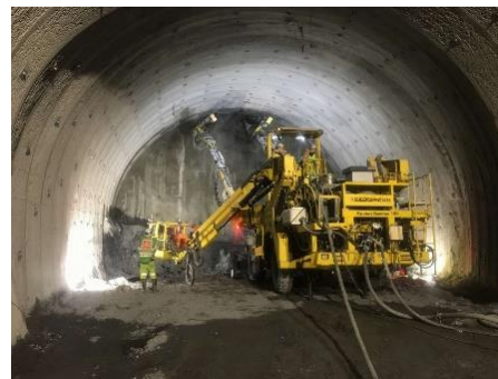
Southern Alps Tunnel Nagano Section Excavation of main tunnel
