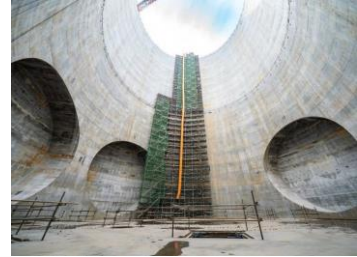
Kajigaya Emergency Exit
