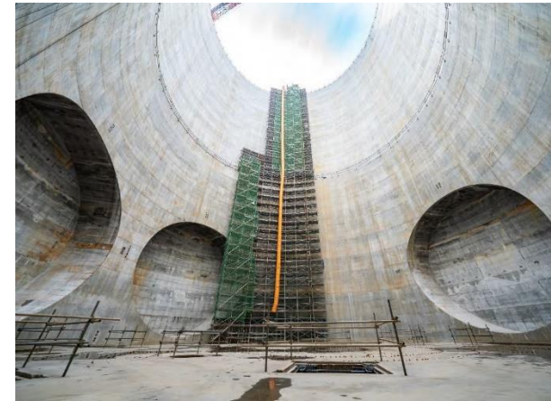
Kajigaya Emergency Exit
