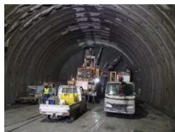
Ina Sanchi Tunnel (Aoki River Section)
