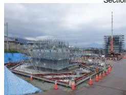
Elevated bridge in Yamanashi Prefecture
