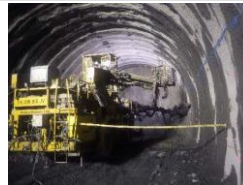
Southern Alps Tunnel (Yamanashi Section)
