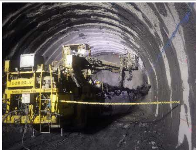
Southern Alps Tunnel (Yamanashi Section)
