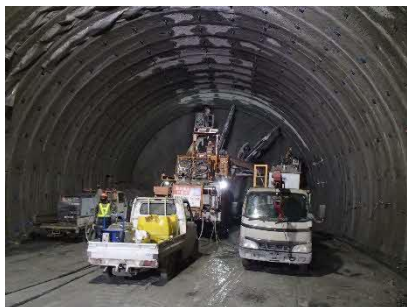
Ina Sanchi Tunnel (Aoki River Section)
