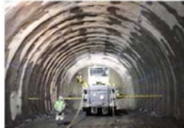
Southern Alps Tunnel (Yamanashi section)
