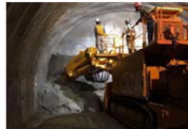
Hiyoshi Tunnel (Minamigaito section)
