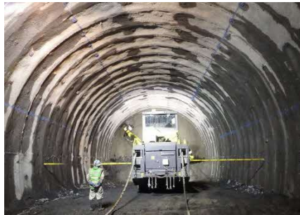
Southern Alps Tunnel (Yamanashi section)
