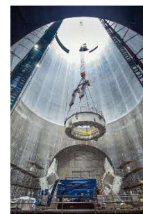
North Shinjima Emergency Access
