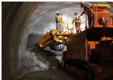
Hiyoshi Tunnel (Minamigaito section)
