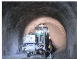
Southern Alps Tunnel (Nagano section)
