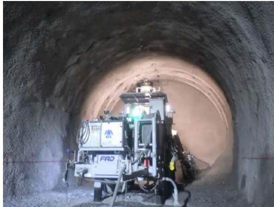
Southern Alps Tunnel (Nagano section)
