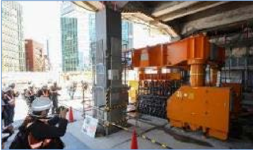
Shinkansen section: Building of the underground diaphragm walls
