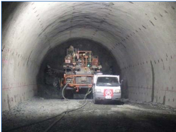
Drilling of inclined shaft
