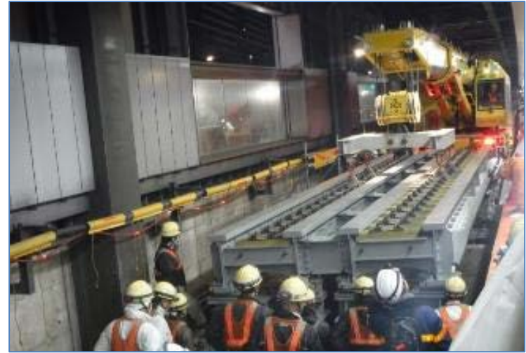
Erection of construction beam
