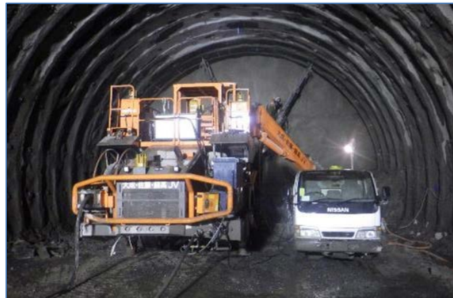
Drilling of main pit
