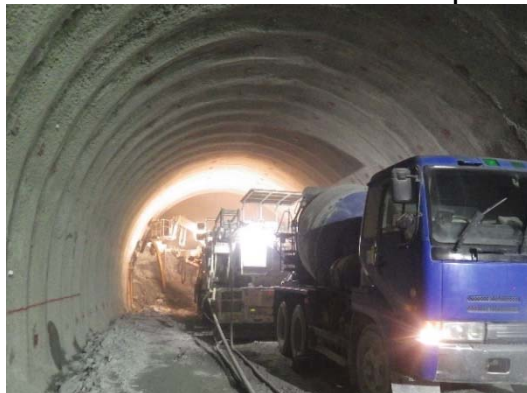
Inclined shaft excavation at the Southern Alps tunnel (Nagano Section)
