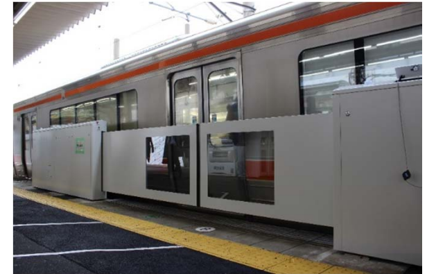
Movable platform fences undergoing verification testing at Kanayama Station
