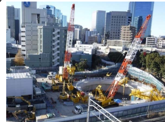
Shaft excavation at Kita-Shinagawa emergency exit
