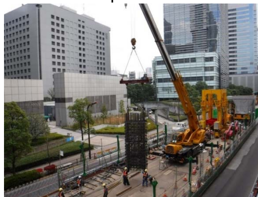
Diaphragm wall construction at Shinagawa Station
