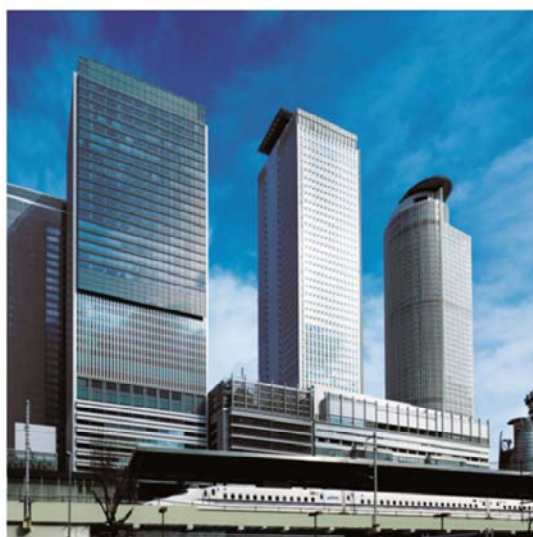
JR Gate Tower (left) and JR Central Towers (center, right)
