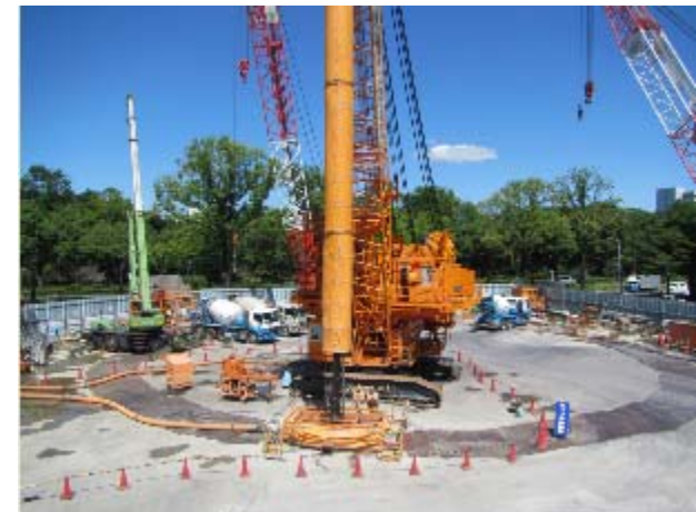
Meijo emergency exit (Diaphragm wall work)
