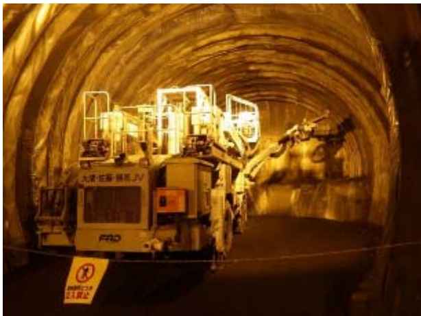
Southern Alps tunnel (Yamanashi section) (Pilot tunnel excavation)
