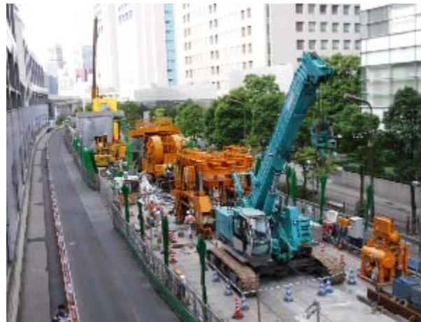
Shinagawa Station (Diaphragm wall work in underground station)
