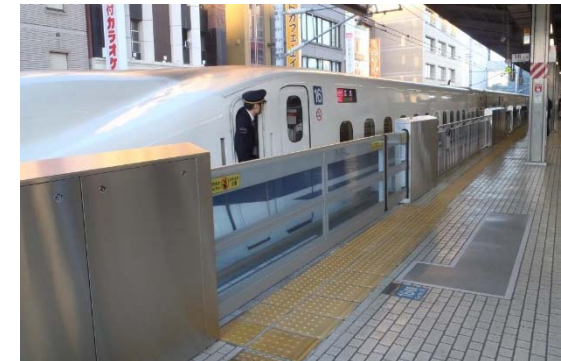
Movable platform fences (Nagoya Station)
