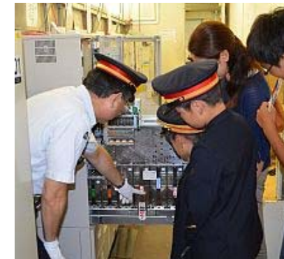
Experiencing work at a station (sample illustration)
