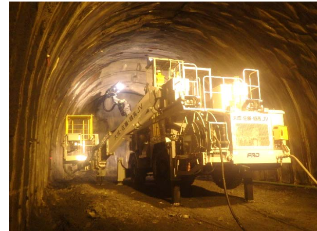
Construction of the Southern Alps tunnel (Yamanashi section)
