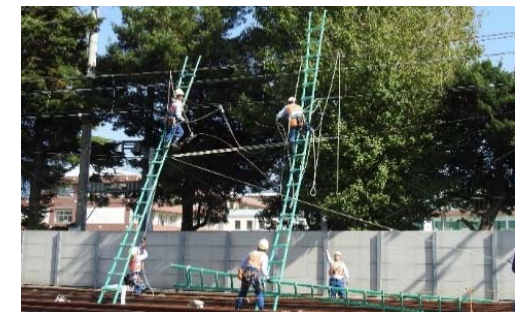
Training for recovering disconnected overhead contact lines
