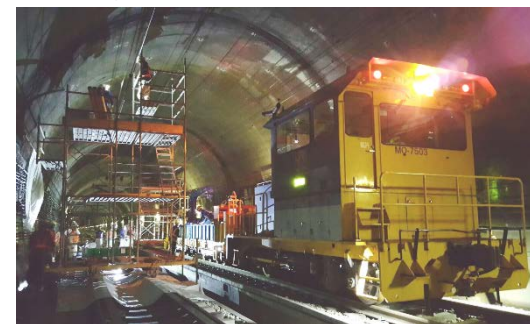
Large-scale renovation (tunnels)
