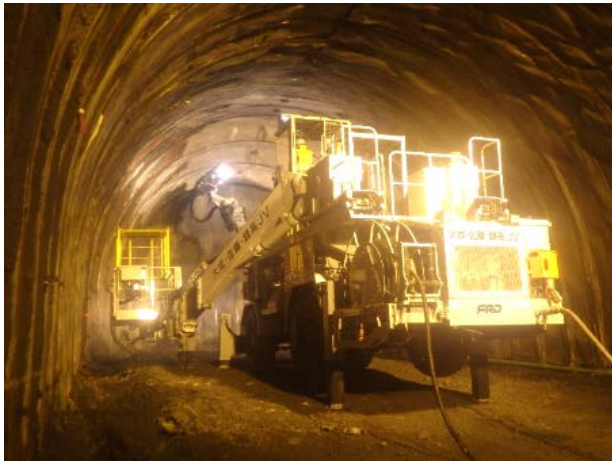
Southern Alps Tunnel (Yamanashi construction section)
