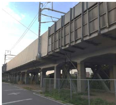
Large-scale renovation (concrete bridges)
