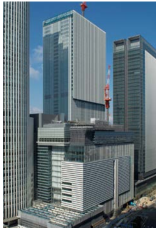
“JR Gate Tower” appearance (photo taken March 2016)
