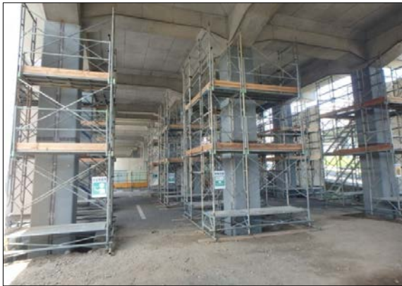
Making conventional line elevated track columns quake-resistant (steel plate jacketing method)
