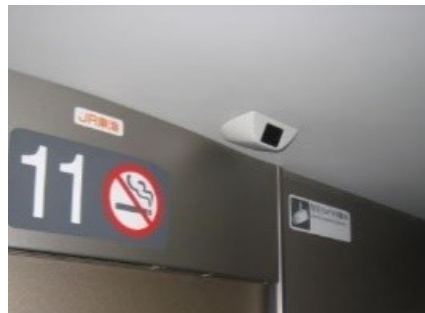
Security cameras (image installed in deck)
