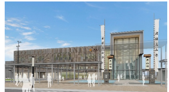
Completed image of Takayama Station
