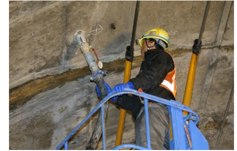
Large-scale renovation (for tunnel/ grout injection behind lining)
