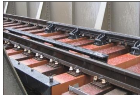
Derailment prevention guards (for non-ballast bridges)
