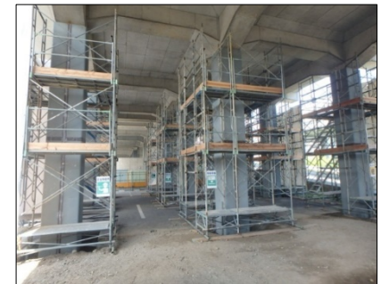
Making conventional line elevated track columns earthquake-resistant (steel plate jacking method)
