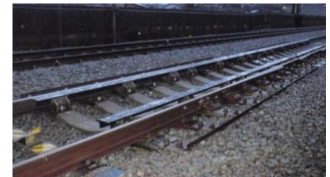
Derailment prevention guards (for expansion joints)
