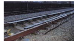
Derailment prevention guards (for expansion joints)
