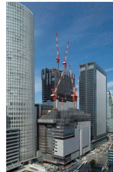
Construction of “JR Gate Tower” (as of September 29, 2015)
