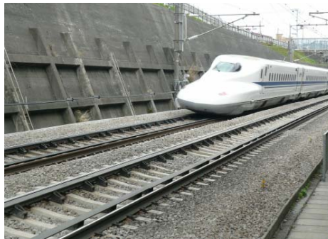
Derailment Prevention Guards
