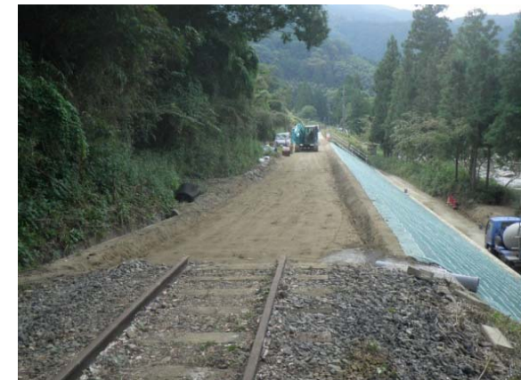
Meishō Line Repair Work
