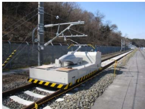
Contact Line Test Installation
