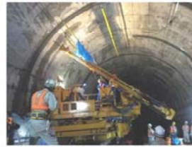
Large-Scale Renovation (Installing rock bolts in inner wall of tunnel)
