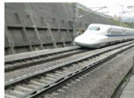
Derailment Prevention Guards
