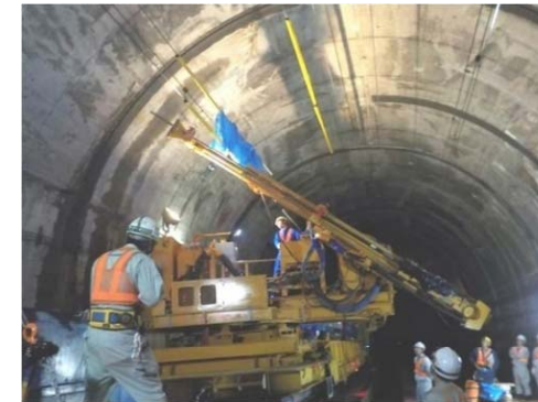
Large-Scale Renovation (Installing rock bolts in inner wall of tunnel)
