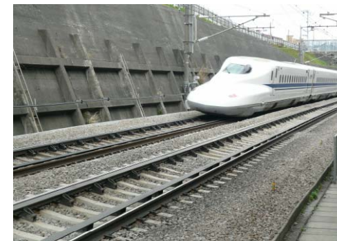
Derailment Prevention Guards
